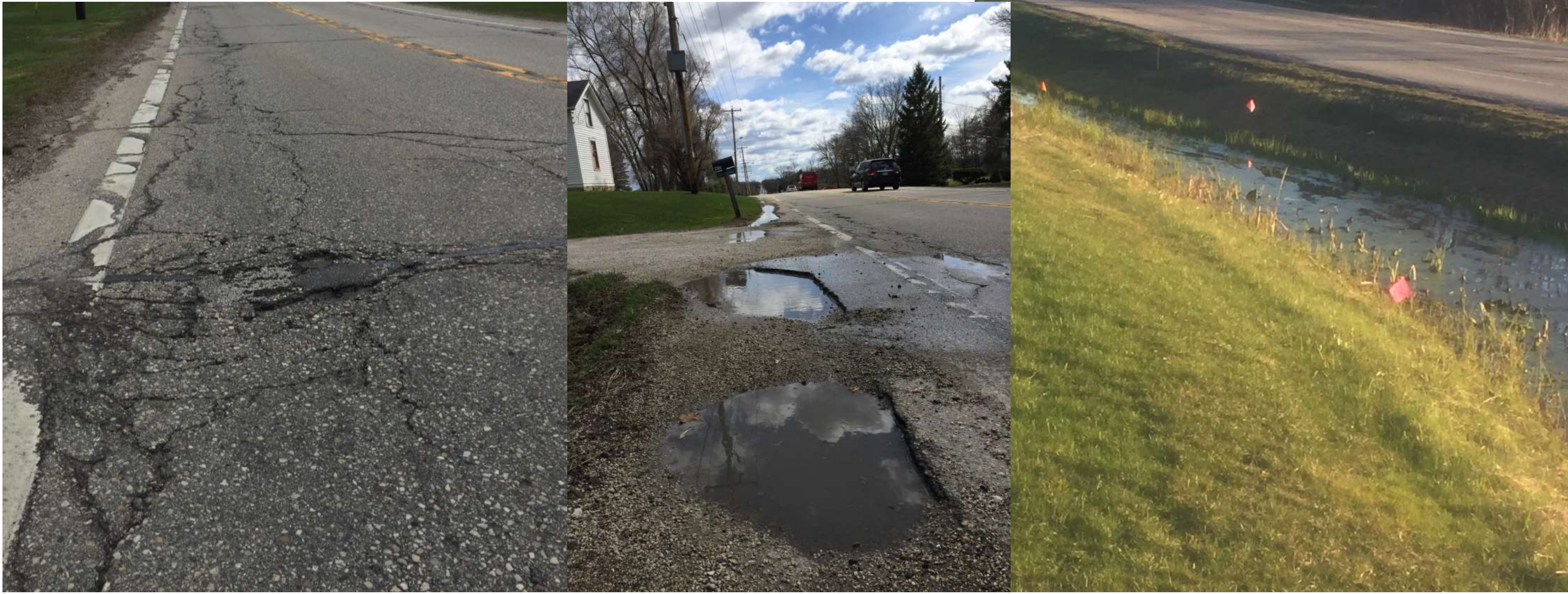
Deteriorated Pavement, Potholes, and Poor Roadside Drainage
